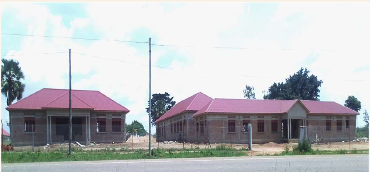
Front view of Maracha Chief Magistrates Court Buildings
