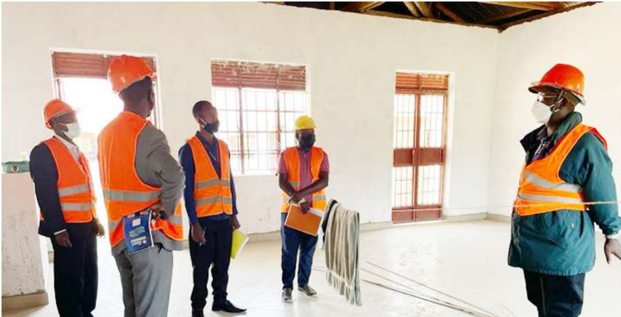
PS/SJ inspecting the construction of Kamwenge Court
